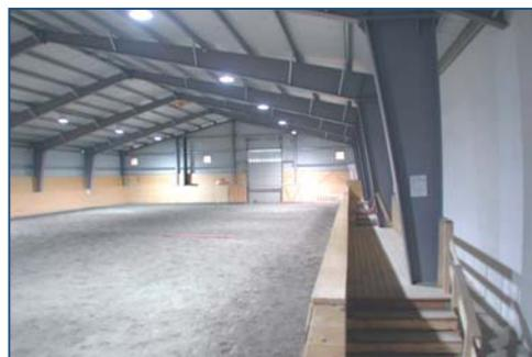
This center located in Hammerfest (N), the most Northerly city in the world, was built during winter 2002/2003 by Builder Naeringsbygg AS. It is designed to resist the extremely high wind and snow loads of this polar area.
