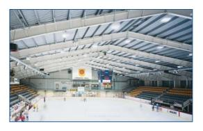
Lørenskog (N) is a ice hockey stade, built in 1987 by builder Gunnar M. Backe. Type: AS 50m span, eave height: 9.10m Surface: 3,350 m<sup>2</sup>
