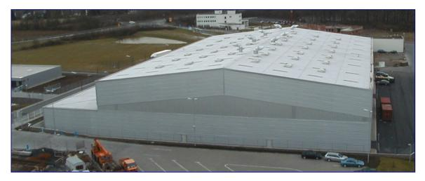
Spanish company LamiGraf ordered this production building for its German branch office in Bönen (D) via local ASTRON Builder ACIEROID. The building is noteable for its impressive 60m free span and was specially designed for the installation of paper coating machines. Annexes to the main structure accomodate the offices and the social rooms. Total floorspace is 7,500 m<sup>2</sup>.
