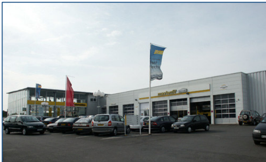
SCI Opel in Cormontreuil (F), built in 1999 by C.I.R., architect: B. Nicolas Surface: 2,691 m 2 Type: AZM1/AP Wall system: Eurotec Roof system : PR Span: 45m
