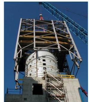
This 24m high, 170 ton structure was built for PRIMOREC Differdange (L). It was assembled on the ground and later lowered over the furnace in a spectacular lift in the summer of 2002.
