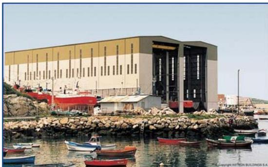
This shipyard was built by builder Agalia in Spain and has a peak height of 28m. There are two internal bridge cranes.
