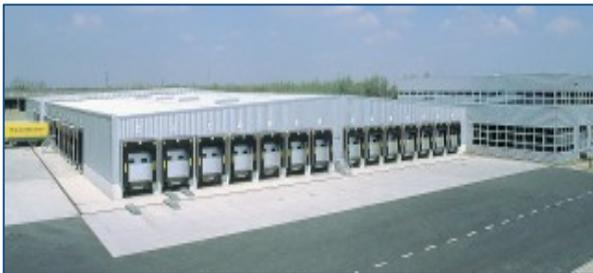
This modern 7,200 m<sup>2</sup> facility was built in Boom (B) by Builder IPES on 13m long piles which were necessary to stabilize the structure on soft clay ground conditions.
