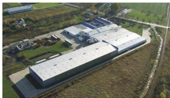
Built by long term builder/dealer Asenhajmer in his home town Elblag/Poland, this furniture plant was several times extended between 1997 and 2006 from AZM-1, span: 26m up to AZM-3, span: 80 m. It has now grown to a total surface of 60,000 m<sup>2</sup>.
