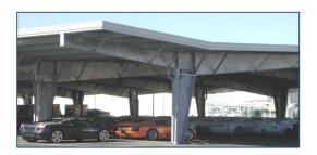
Ruggerini built a special canopy for Lamborghini in Bologna (Italy) to protect finished vehicles stored on the parking area next to the production plant. This AZM1 covers 2,700 m<sup>2</sup> and has a free span of 34 m.
