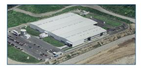
Automotive parts supplier Faurecia built this 11,000 m<sup>2</sup> plant in Vigo (Spain) in 2002. In the past 20 years, 15 factories in Europe come from ASTRON. The company produces seating, exhaust systems, doors and other components for various car manufacturers inside the large 36m clear span AZM1.
